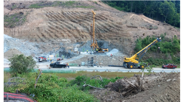
Bridges over New England Road drilled shaft caisson construction.
