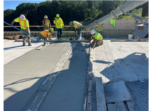
Concrete placement for expansion dam - bridge over Camp Hollow Road.
