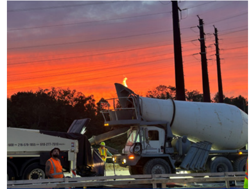
Concrete deck placement - bridge over Camp Hollow Road.
