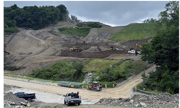
Excavation for bridge construction at New England Road.
