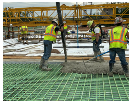
Concrete bridge deck placement - bridge over New England Road.
