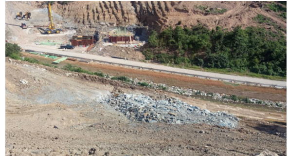
Bridges over New England Road construction progress.
