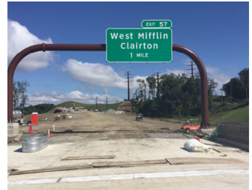
Overhead directional sign installed.
