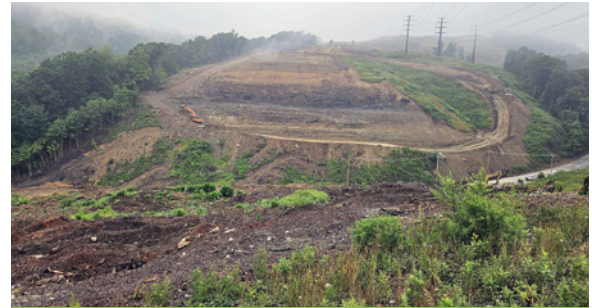
Excavation for bridges over Camp Hollow Road.
