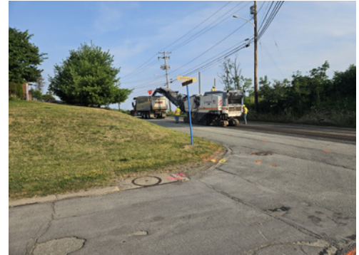
Milling existing Old Camp Hollow Road to repave.
