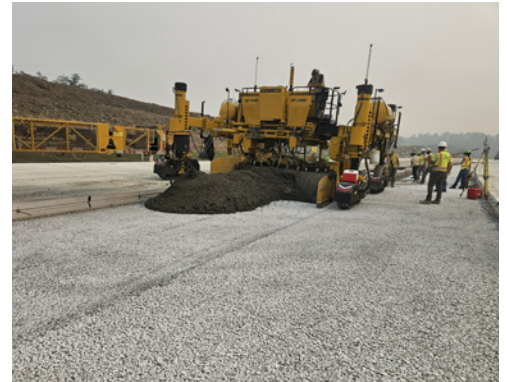
Median shoulder concrete paving.
