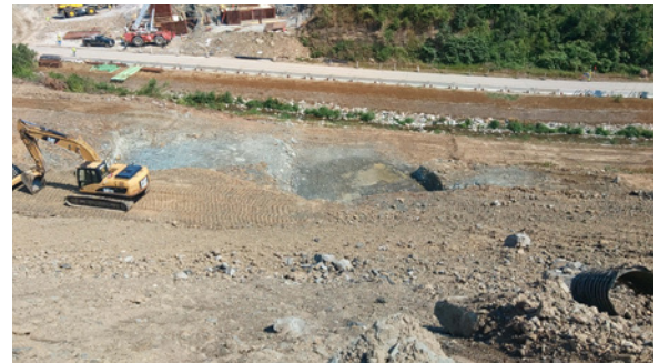
MF-406-407 Pier-2 excavation (bridges over New England Road).
