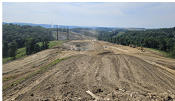
Sediment basin construction.
