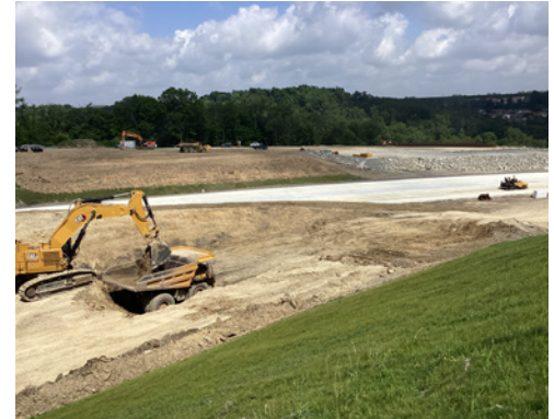
Northbound on ramp excavation for future Camp Hollow Road interchange.
