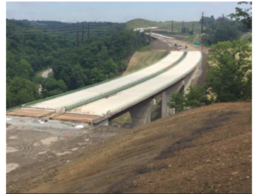
Bridges over New England Road - construction progress.
