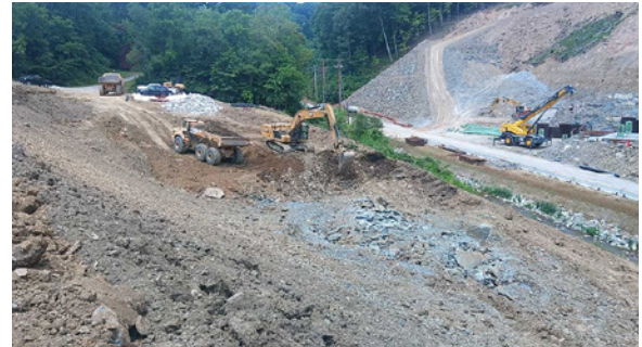
Excavation work at Pier 2 where bridges will span New England Road.
