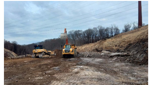
Excavation for bridge abutment at Camp Hollow Road.
