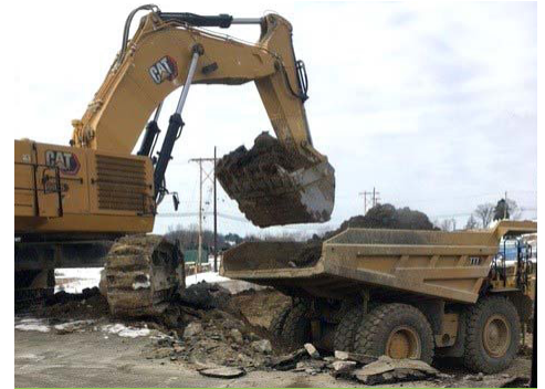
Excavation near Camp Hollow Road field office.
