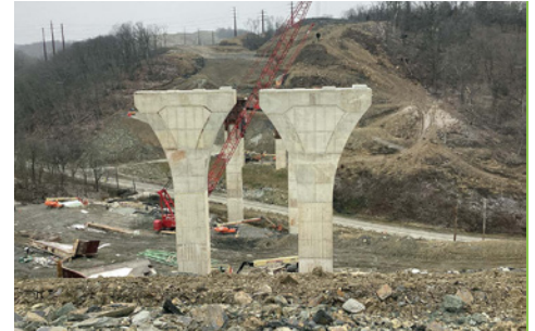
Construction of bridge piers over New England Road.
