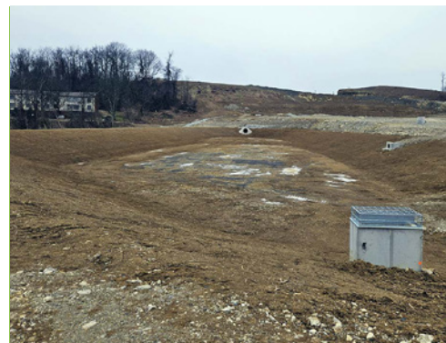
Sediment basin built near Curry Hollow Road.
