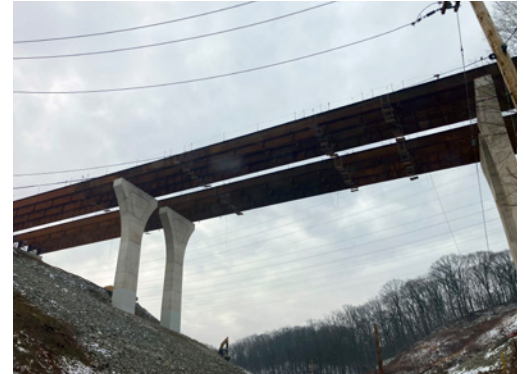
Bridges over Camp Hollow Road - steel girder installation complete.
