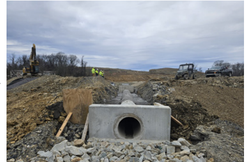
Stormwater drainage pipe installation.
