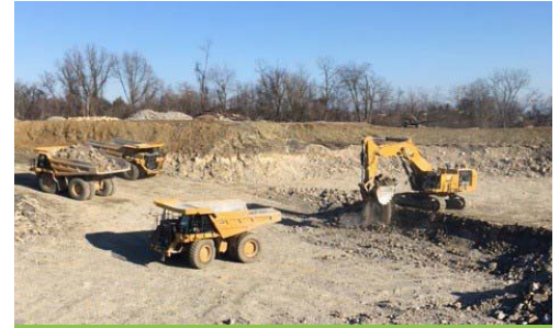
Camp Hollow excavation- roundabout area.
