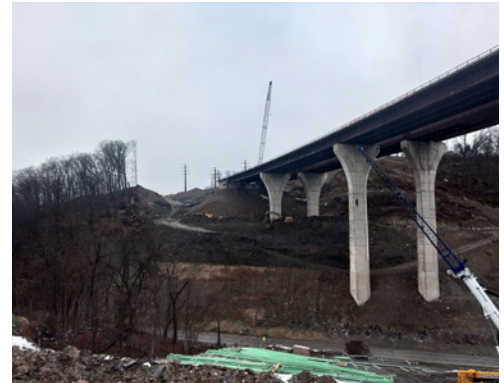
Bridges over New England Road - construction progress.
