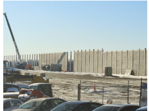
Soundwall - construction progress.
