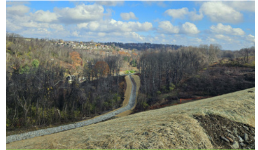
Completed Stream Relocation Near Curry Hollow Road.
