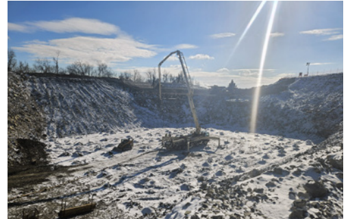
Mine grouting for future Camp Hollow interchange bridge.
