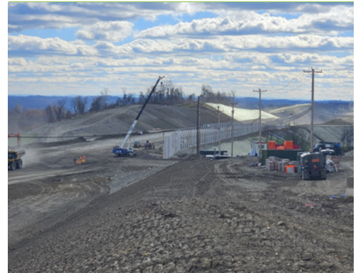
Sound wall construction along new alignment.
