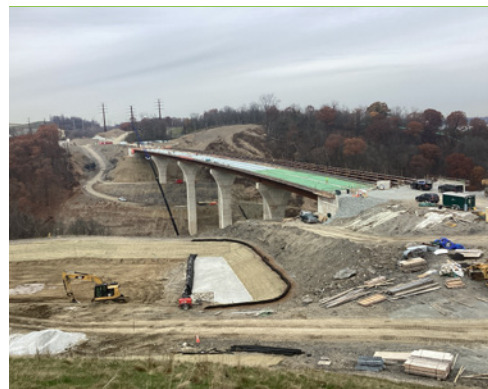
Bridges over New England Road - construction progress.
