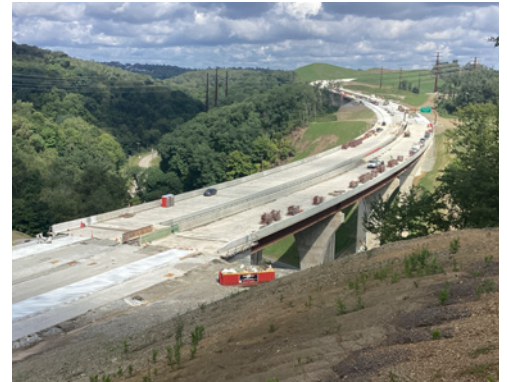
Bridges over New England Road - construction progress.
