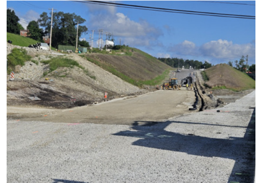
Southbound on ramp at Camp Hollow Road - construction progress.
