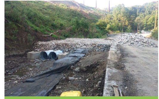
Temporary stream crossing from Camp Hollow Road.
