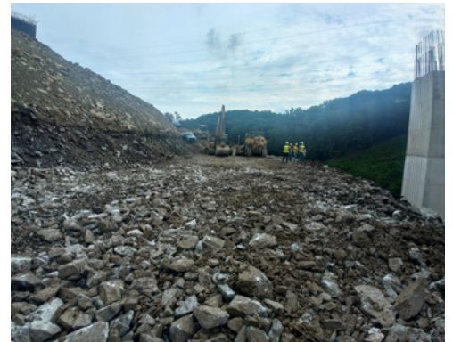
Constructing crane pad for bridge over New England Road.
