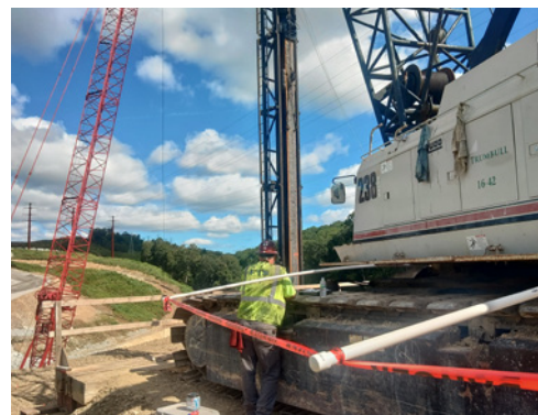
Driving steel H-piles for bridge over Camp Hollow Road.
