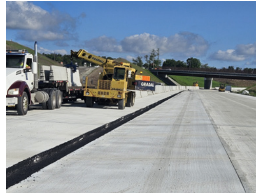
New highway concrete median barrier installation near Camp Hollow Road.
