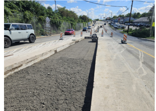
Lebanon Church Road turning lane work.
