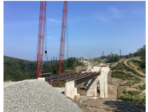
Steel girder installation for bridges over New England Road.
