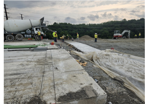
Sleeper slab concrete placement.
