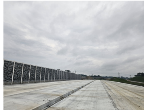
New concrete highway near sound wall at Camp Hollow Road interchange.
