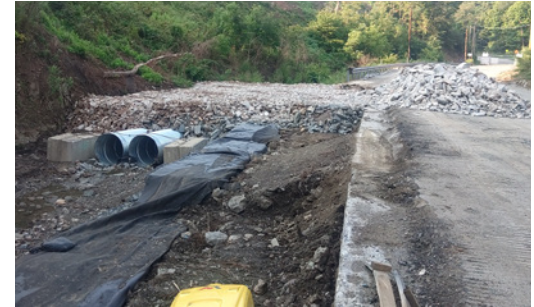
Temporary stream crossing from Camp Hollow Road.
