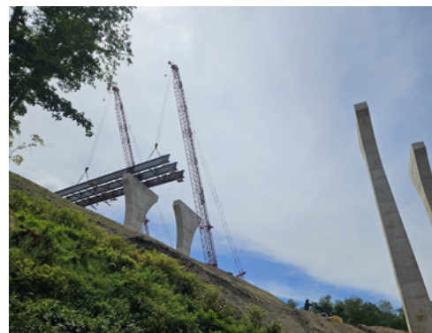
Steel girder installation for bridges over New England Road.
