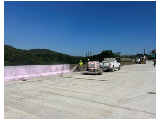
Bridge parapet curing application - bridge over New England Road.
