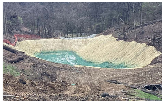
Temporary erosion and sedimentation control measures.
