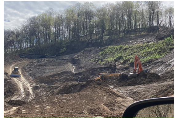
Bridges over New England Road excavation.
