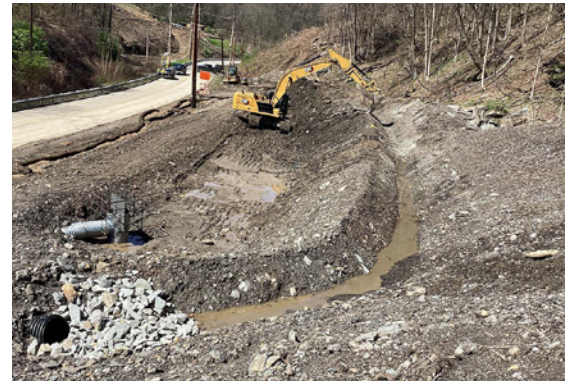
Construction of temporary sediment trap along New England Road.
