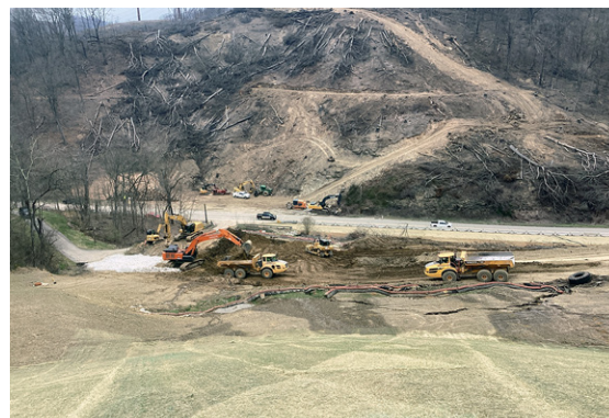
New England Road excavation.
