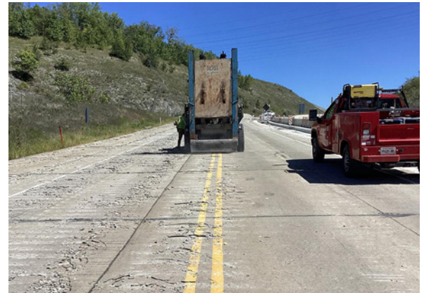
Demo of existing Jefferson Boulevard pavement.
