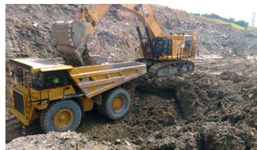
Bulk excavation occurring near Jefferson Blvd.
