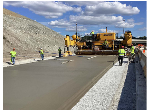
Concrete paving for reconstructed Jefferson Boulevard.
