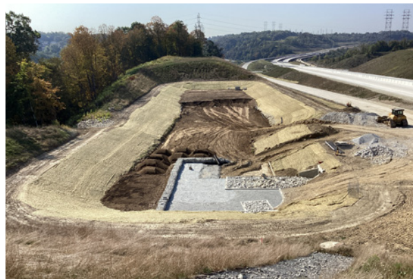
Stormwater management pond construction.
