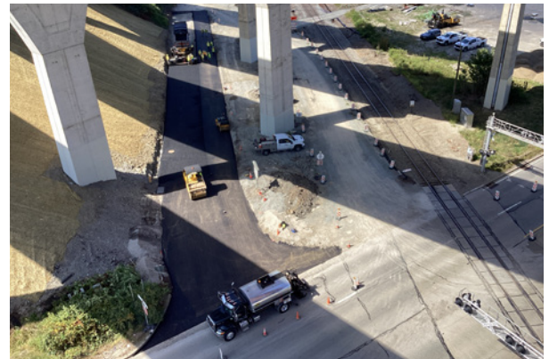
Brickyard Road asphalt paving.
