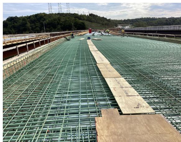
Bridge deck construction for bridges over SR-51.
