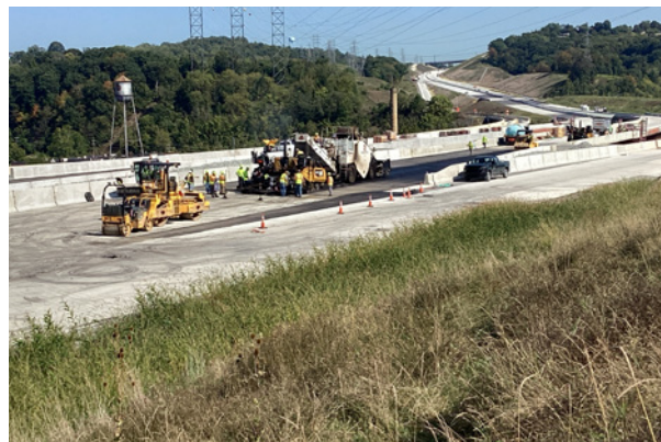
Bridge approach asphalt paving.
