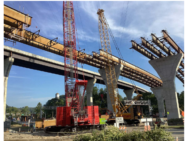
Steel girder installation over SR 51.
