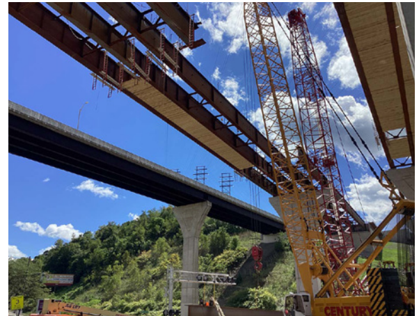
Bridge beams recently placed over SR51.
