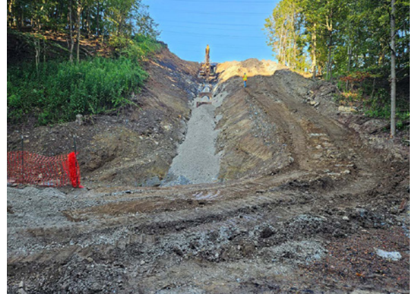
Drainage pipe installation.
