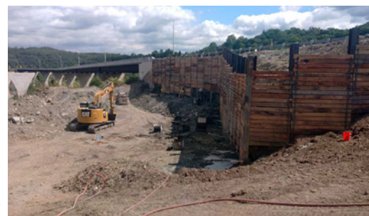
Temporary shoring at the southbound bridge over the SR51 abutment.
