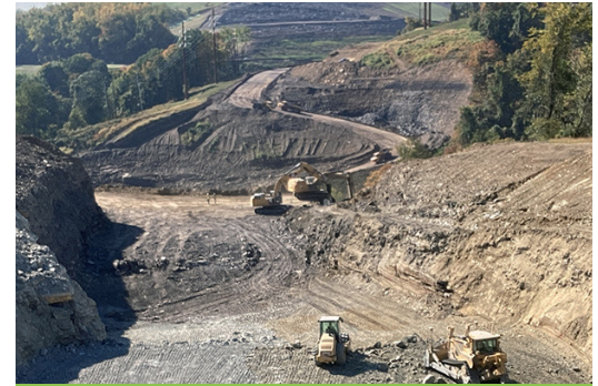
Bulk excavation work throughout the project in Jefferson Hills Borough.
