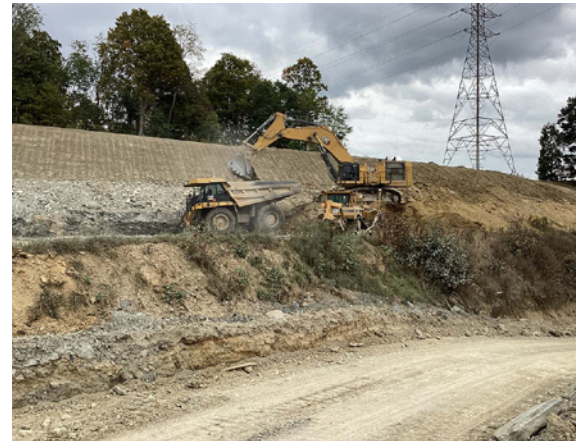
Bulk excavation for new highway alignment near Jefferson Boulevard.
