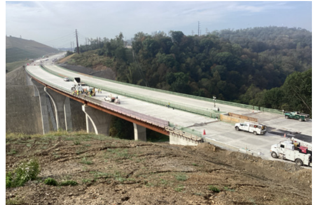
Bridges over Coal Valley Road construction progress.
