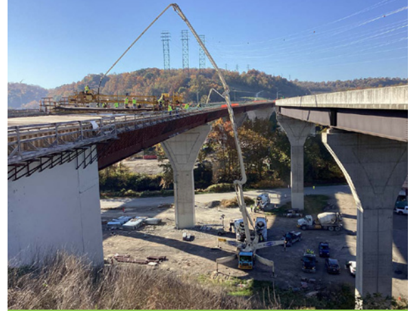
Concrete deck placement for bridges over SR51.
