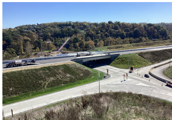
Jefferson Boulevard interchange.
