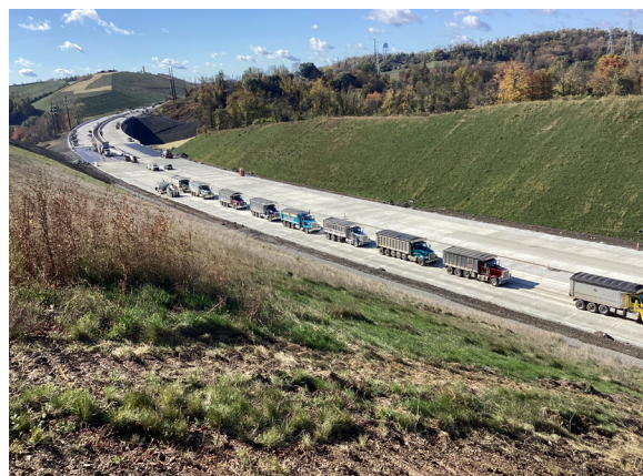
Asphalt bridge transition paving for bridges over Coal Valley Road.
